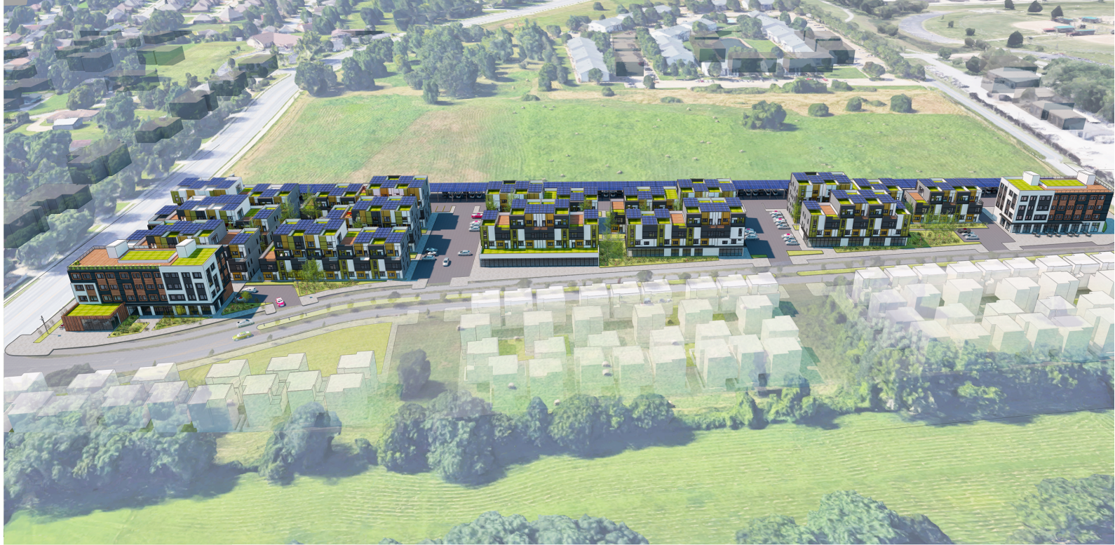
VIEW E: BIRD'S EYE VIEW LOOKING SOUTH
